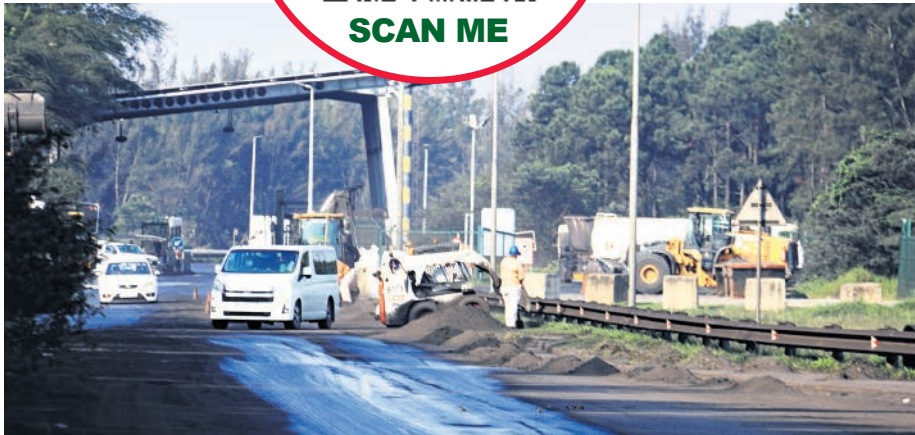
The Port of Richards Bay's east gate has been closed to coal trucks, and rehabilitation work at the access began on Thursday
